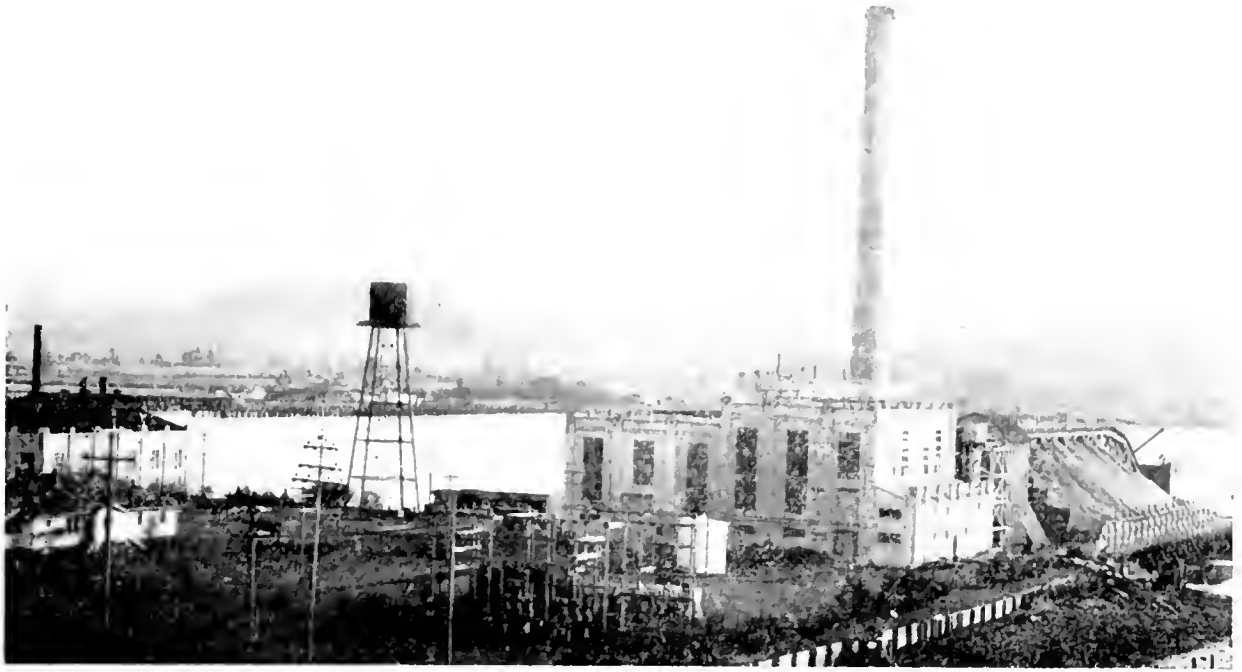
Astoria Steam Generating Station - Built in 1920 by Pacific Power & Light Company
